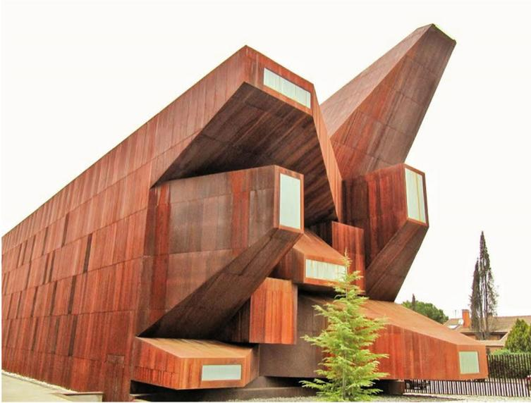
**Fig. 1** Santa Mónica parish in Rivas-Vaciamadrid (Spain) built with Cor-Ten steel. Note the spectacular colour of the patina formed on the steel surface (photo taken by the author)
