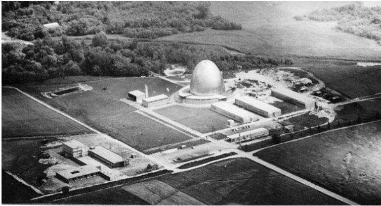
Fig. 1 The site of the Garching research reactor (the egg-shaped building) in about 1960. Mössbauer had set up his laboratory in the left of the two low barracks facing the reactor
